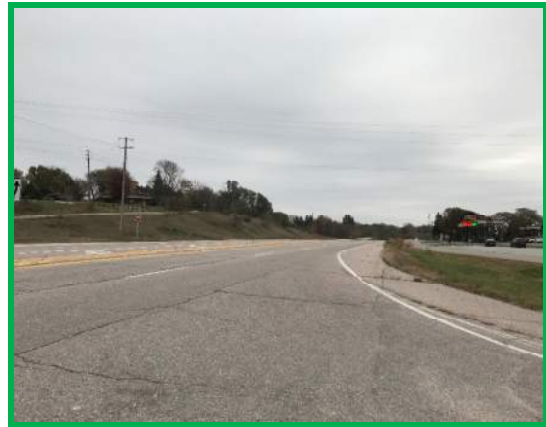
Virginia Hills Rd Looking East at the Intersection
