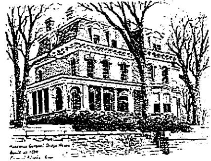
Historic Dodge House: 605 Third Street
