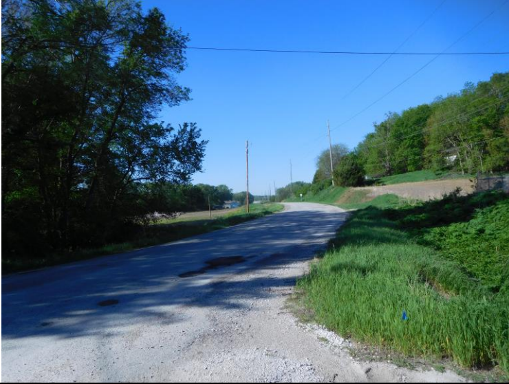
View south along State Orchard Road
