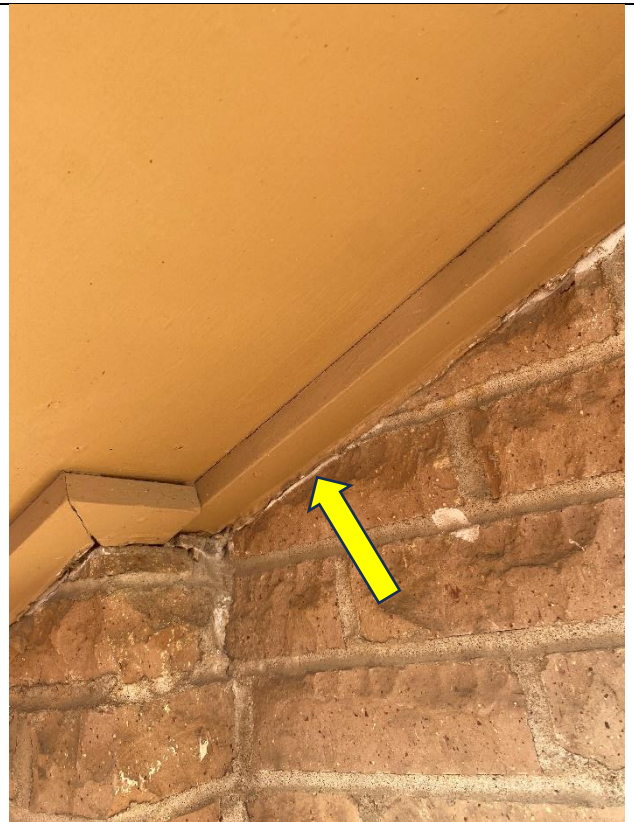
PHOTO 18 HA-019 Soffit caulking / Gray. Non-ACM
