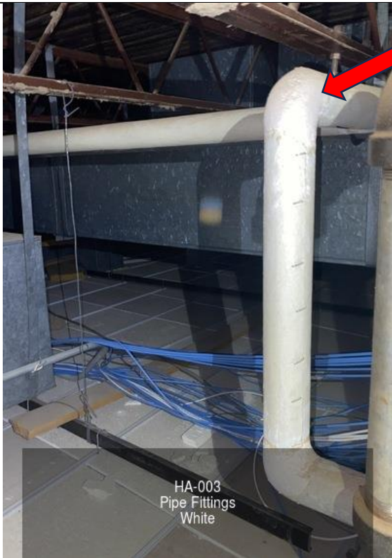
PHOTO 3 <1% Amosite, 3% Chrysotile: 2024 Sampling 3% Amosite, 15% Chrysotile: 2017 Sampling
