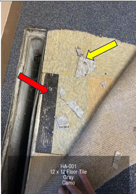
PHOTO 1 Non-ACM 12 x 12 Gray Camo VFT & ACM Black Mastic (2% Chrysotile)
