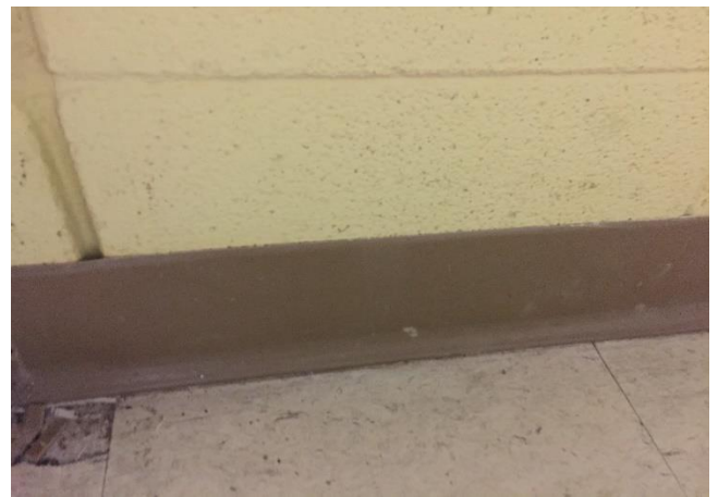
PHOTO 23 Non-asbestos containing 4" brown vinyl wall base HM#: MM-02
