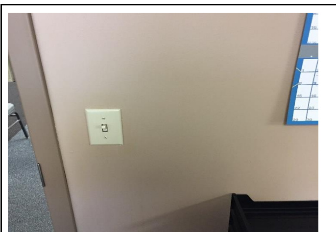
PHOTO 37 Non-asbestos containing drywall and joint compound system. HM#: MM-16
