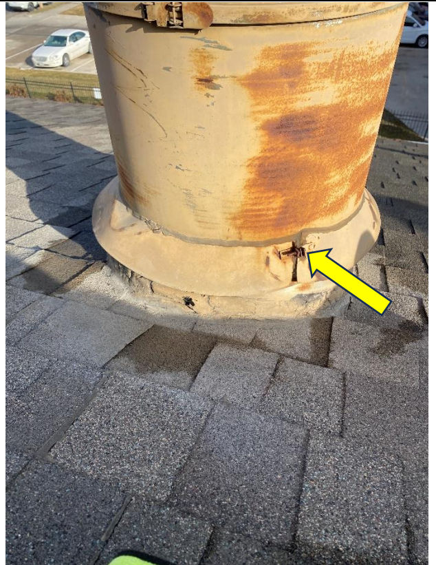
PHOTO 20 HA-021 Exhaust caulking / Black. Non-ACM
