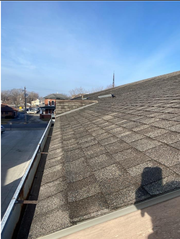
PHOTO 19 HA-020 Roofing Shingles. Non-ACM
