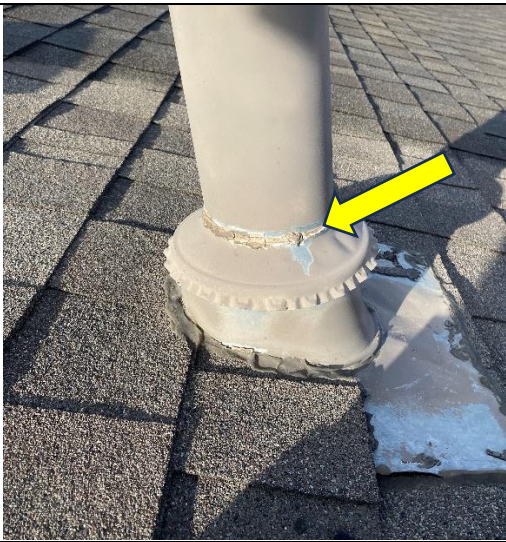
PHOTO 21 HA-022 Exhaust caulking / White. Non-ACM
