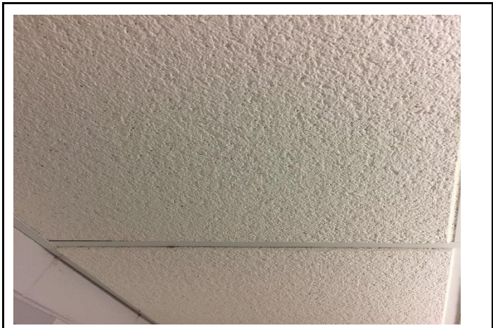
PHOTO 28 Non-asbestos containing 2'x2' ceiling tile. HM#: MM-07
